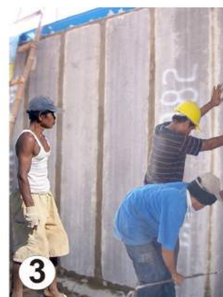
3 joint between pariton wall covered with mortar.
