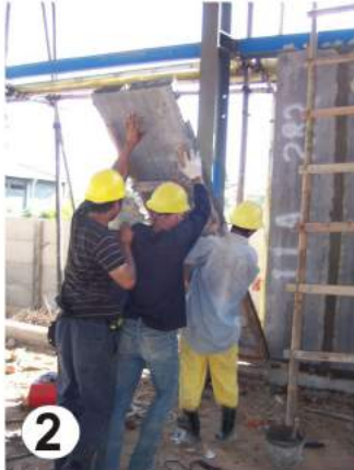
2 procces of installation of pariton wall
